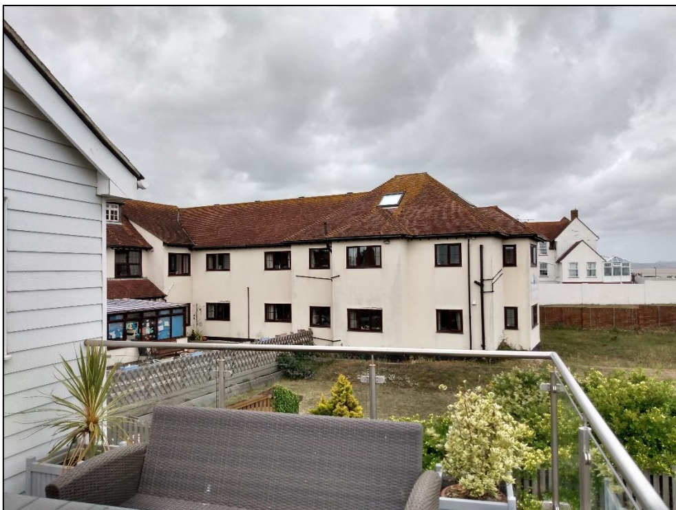
Flank view from balcony of The Coast House (to south)
